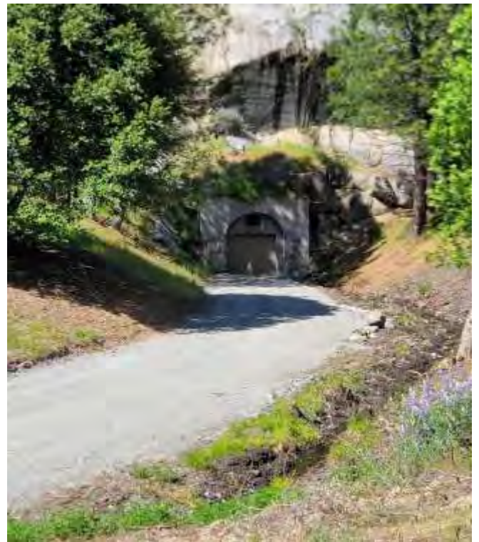
Sandbar Tunnel Access - After
