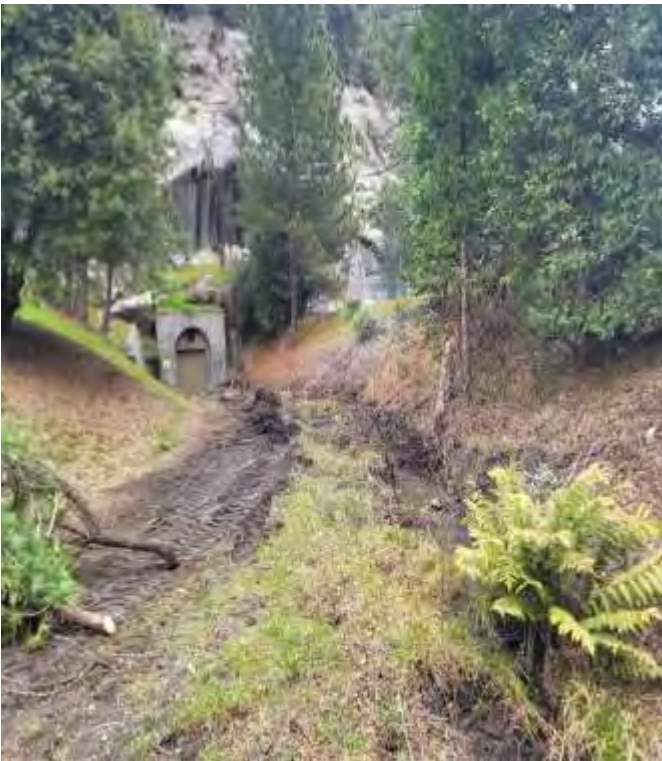
Sandbar Tunnel Access – Before
