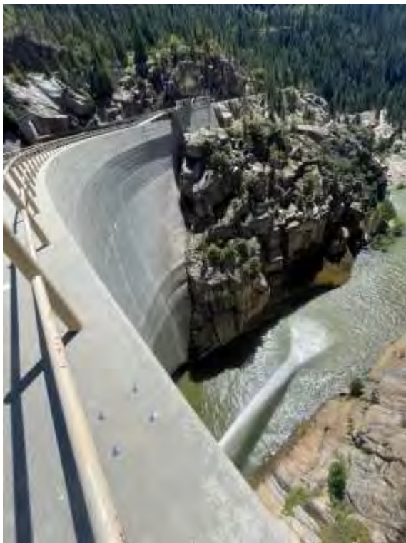
Donnells Vegetation Clearing
