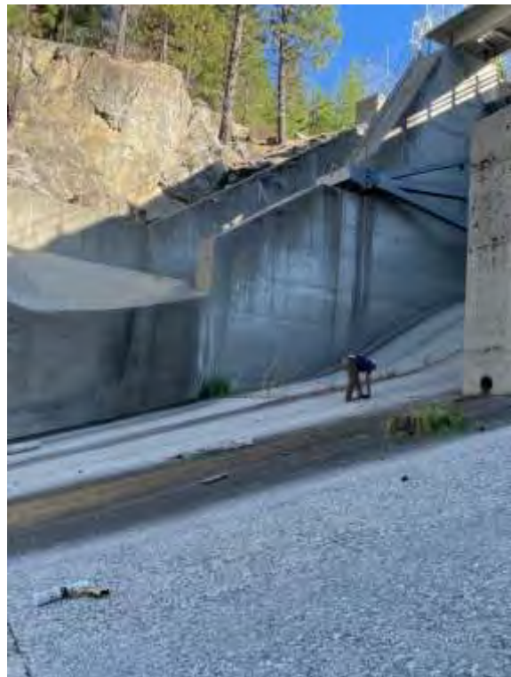
Beardsley Spillway Maintenance
