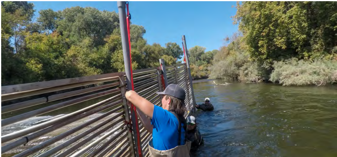
Figure 1. Stanislaus River weir installation.
