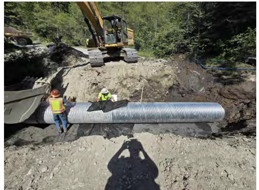
Culvert at Sta 11+13 looking NE
