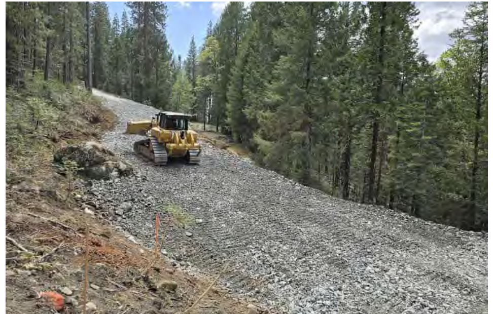
Looking SW from Sta 9+25 cutslope
