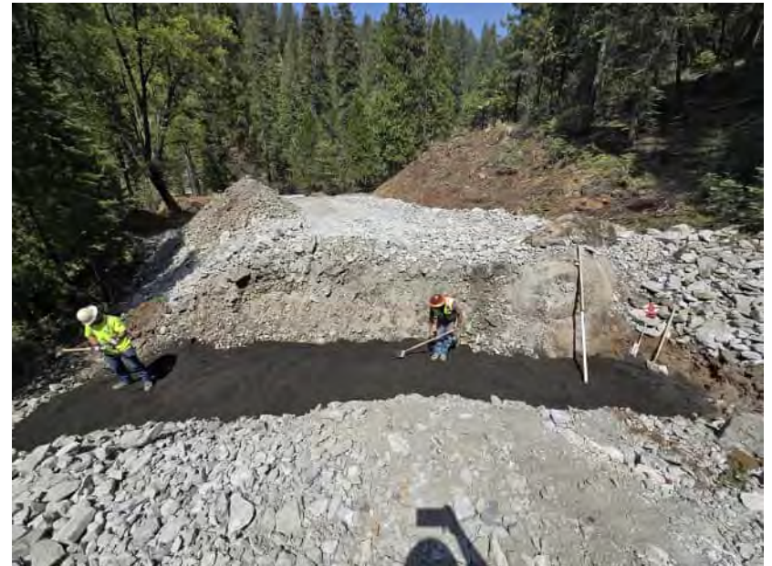
Culvert at Sta 8+00 looking NE
