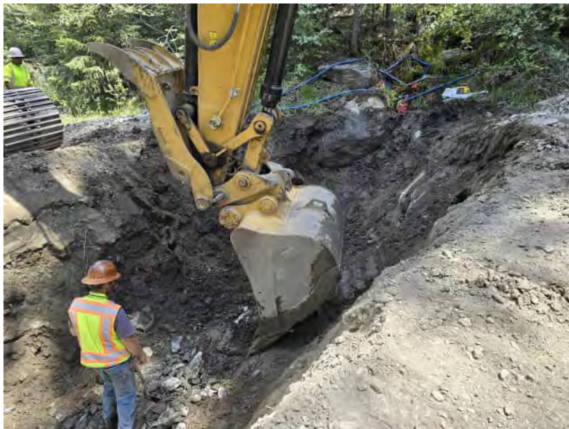
Culvert at Sta 11+13 looking E
